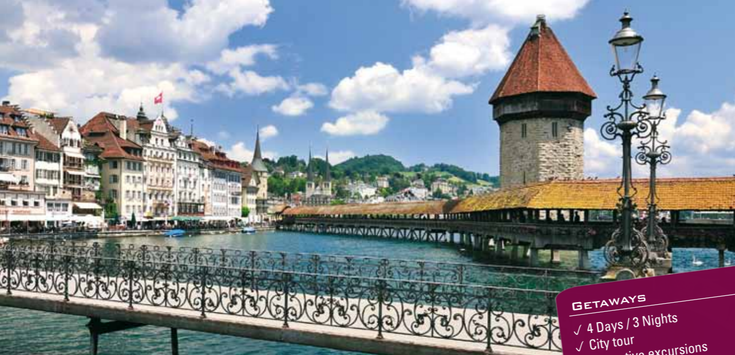
Bridge Kapellbrücke, Lucerne / Switzerland
